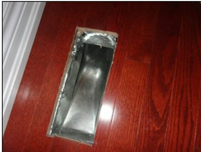
24. There are gaps between heat diffusers, cold...
